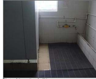
Photo of the sanitary facilities toilet.JPG
