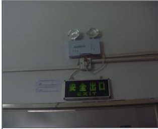
Photo of fire safety equipment exit with emergency light and exit sign.JPG
